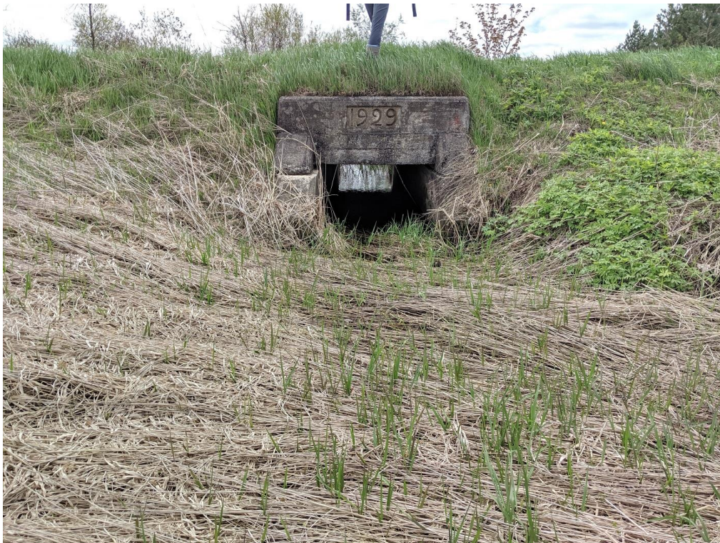
Photograph 2: East box culvert beneath the rail corridor (May 24, 2019).
