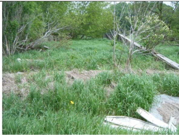
PLATE 3 RUINS WITH CONCRETE FOUNDATION
