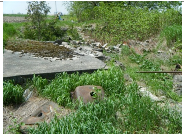
PLATE 2 RUINS WITH CONCRETE FOUNDATION
