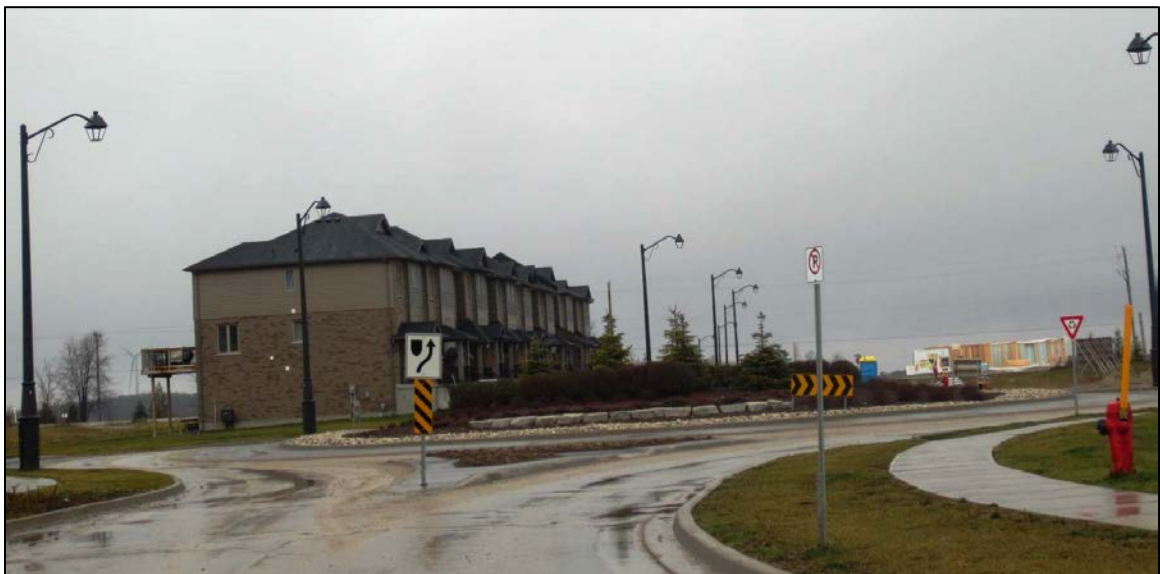
Figure 23: Roundabout at Taylor Drive / Mill Street
